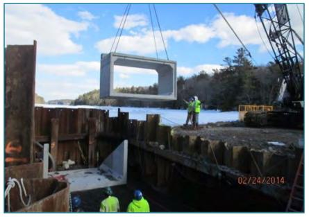
FIGURE B.8 - Maine DOT installation of precast concrete box culvert with twelve-foot span and six-foot rise. Long Reach Lane, Long Marsh, Harpswell, ME. Image source: Casco Bay Estuary Partnership.
