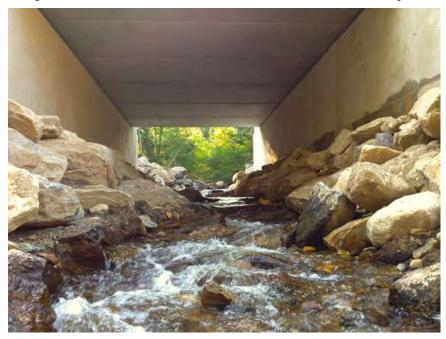
FIGURE 5.3 - This MaineDOT crossing was designed to adequately accommodate storm flows, protect footings from scour, facilitate low-flow water depths sufficient for fish passage, and allow for semi-aquatic wildlife movements. Photo by Slade Moore.
