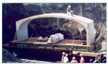
FIGURE B.9 - A three-sided rigid frame section. Image source: Precast Solutions.
