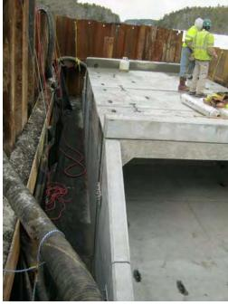
FIGURE 8.2 - A sheetpile coffer dam was utilized to isolate the work area from tidal flows during the replacement of the Long Reach Lane tidal crossing in Harpswell. Photo by Charlie Hebson
