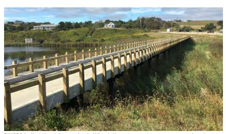
FIGURE B.2 - Single-lane bridge on piers in Chilmark, Massachusetts, that spans an area projected to flood more frequently with sea level rise. Photo by Slade Moore.
