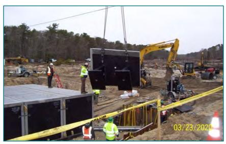
FIGURE B.11 - A pre-cast wingwall installation for a three-sided rigid frame with pre-cast footings. Coonamessett River, Falmouth, MA. Image source: Chris Bennett.
