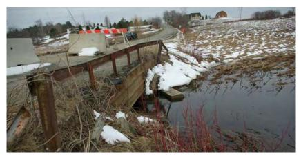
FIGURE 1.14 - Like many aging crossings, this one was replaced well after its safe, useful service life concluded. Photo by Slade Moore.
