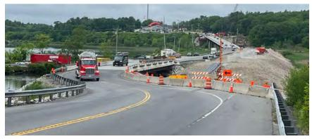
FIGURE 8.1 - When tidal crossings are replaced in primary traffic corridors, temporary traffic bypasses may be required. This temporary bypass along Route 1 in Woolwich, Maine, was used during bridge replacement and construction to restore tidal flow to Back River Creek Marsh. Photo by Michael Burke.
