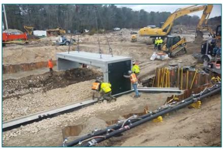
FIGURE B.10 - A three-sided rigid frame section being installed on pre-cast footings. Coonamessett River, Falmouth, MA. Image source: Betsy Gladfelter.
