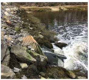
FIGURE 1.8 - This perched, undersized culvert blocks aquatic organism passage except during high tide. Photo by Slade Moore.
