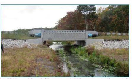
FIGURE B.6- A three-sided concrete rigid frame structure, installed on pre-cast footings. Clear span of 24 feet. Structure includes a pre-cast modular design with six-foot-long sections. Due to cover limitations within the road prism, an insulated water line was attached to side of headwall. Coonamessett River, Falmouth, MA. Image source: Inter-Fluve.
