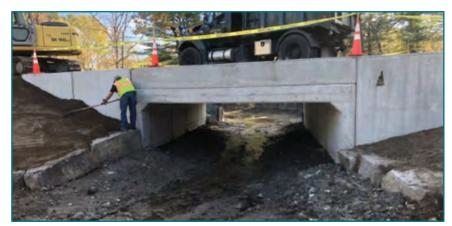
FIGURE B.5 - An embedded pre-cast concrete box culvert, with 16-foot span by 8.5-foot rise. Lubberland Creek, Newmarket, NH. Image source: Peter Steckler.
